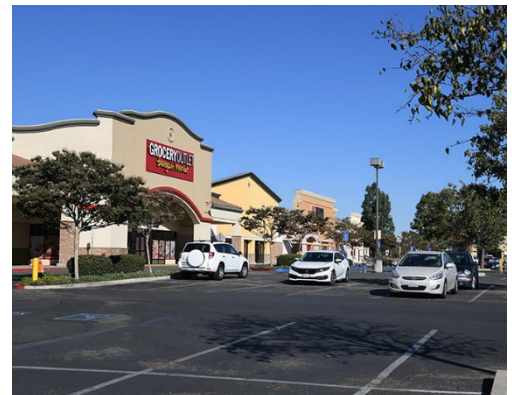
SITE 3A EXISTING CONDITIONS
