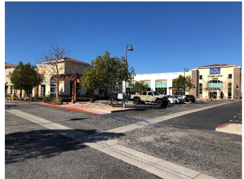
SITE 7 EXISTING CONDITIONS
